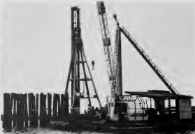
A NEW dolphin is going up in the harbor near the entrance, to be put in use sometime next month. The idea is to relieve dock congestion by berthing ships on the dolphin if they have minor repairs or are taking on bunkers.
